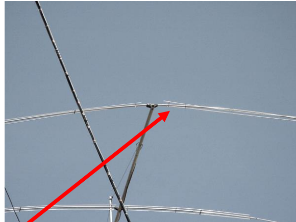
Rectification at unintended, corroded junctions
