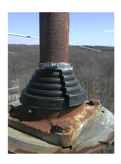
It can also keep the water out of an Orion 2800's top bearing.
