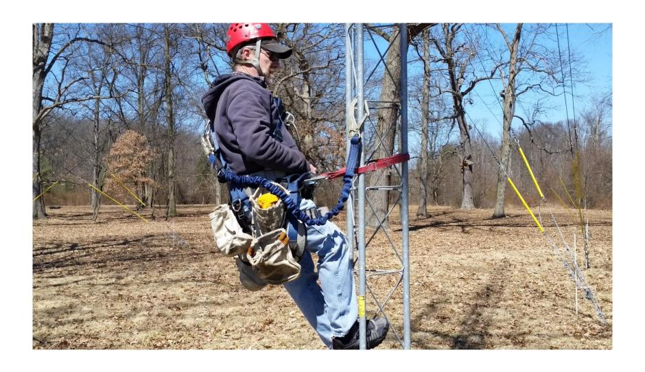
Even if you will not be using a fall arrest lanyard, a full-body harness aids in rescuing you from the tower should that become necessary.
