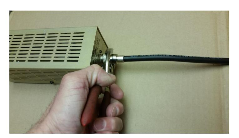
One wrap of 88 tape. And always cut the end when taping. Never pull/tear the end or you'll end up with a tail.
