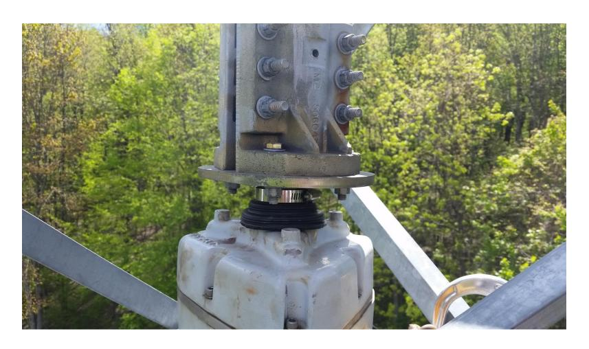
The bolts in a TB3 can seize up. Apply antiseize before installation or swap out the bolts with stainless (and maybe still use anti-seize?)
