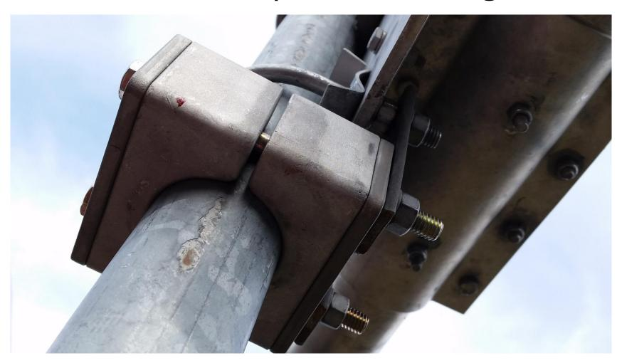
If the top section of your tower is above the top set of guys, the leg bolts MUST be tight and should be regularly checked. This is a point of great lateral stress and if the bolts loosen, the holes in the legs will elongate.
