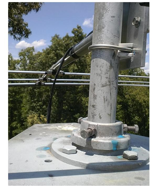
Notice all the blue stuff? You should also use a lubricant on all stainless hardware. Blue Locktite is a good choice. It lubricates, locks, yet can still be removed later.
