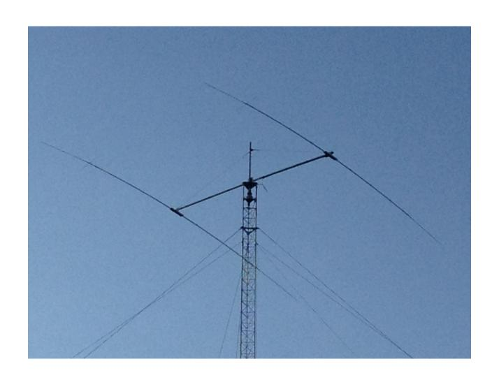
Do not over tighten anything on a Rohn tower leg. You could smash the leg (it can even split) and the tower will be compromised.
